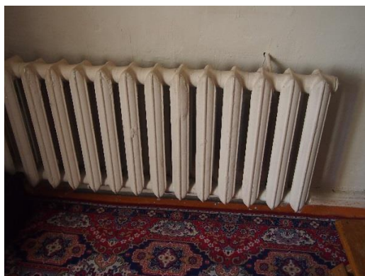
a. Cast iron radiator
