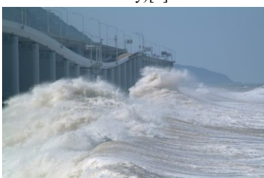
Fig. 1.6 RC bridge in coastal zone attacked by sea waves in winter[5]
