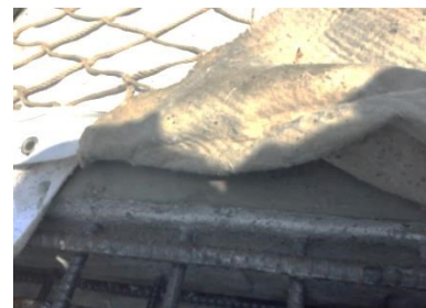
Fig.4.24(i) 28 days wet curing of Kosano RC slab
