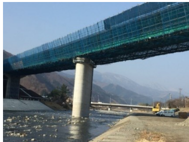
Fig.4.24(b) Kosano Viaduct at Kamaishi, Iwate Prefecture
