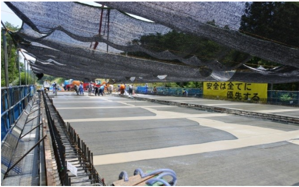
Fig.4.34(b) Providing shades for preventing solar radiation upon newly placed concrete.
