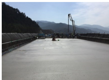
Fig.4.24(h) Finished surface of Kosano RC slab
