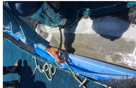
Fig.4.4(b) Continued wet curing under curing mats
