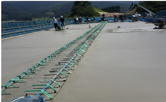
Fig.1.23 Multiple protection highly durable concrete placement
