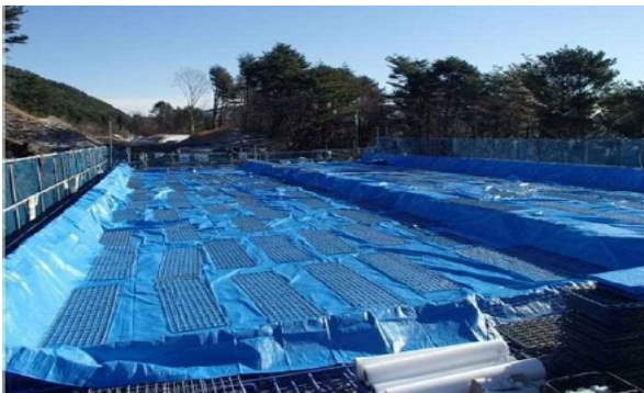
Fig.4.34(d) 28 days wet curing with double layered curing sheets.
