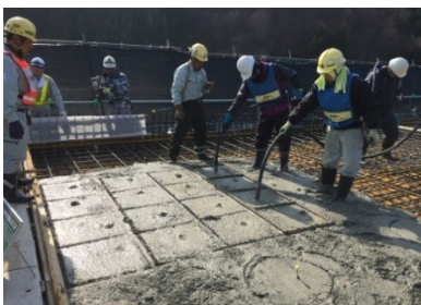
Fig.4.24(g) Durable concrete placing and compaction
