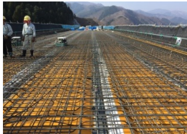
Fig.4.24(e) Steel reinforcement
