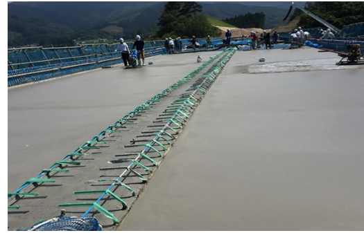
Fig.4.3(b) Placement of durable concrete
