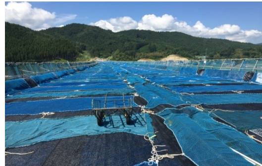
Fig. 1.24 Three layered curing mats for the RC slab
