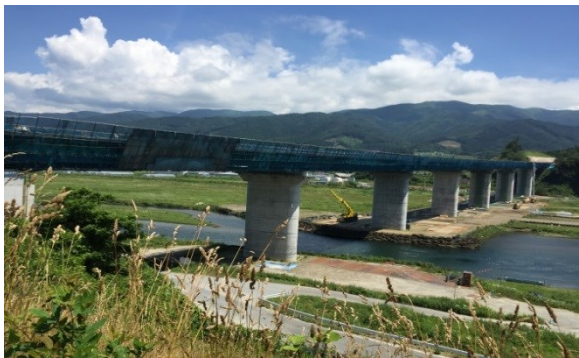
Fig.3.3 (a) Multiple span steel girder Shinkesen Ohashi bridge
