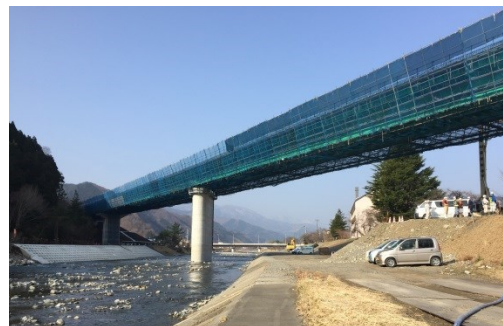
Fig. 1.19 Multiple span Kosano Viaduct, another application of multiple protection durable RC slab in Kamaishi (Length=260m, concrete placement started in March,2018)
