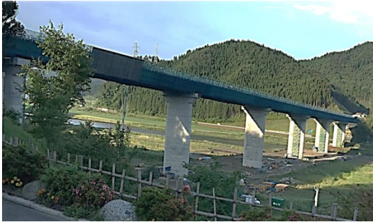
Fig.4.1(a) Shinkesen Ohashi bridge.
