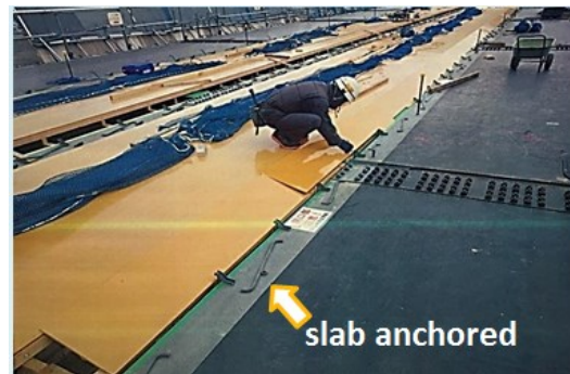
Fig.4.2(b) Slab anchors and mechanical connectors.
