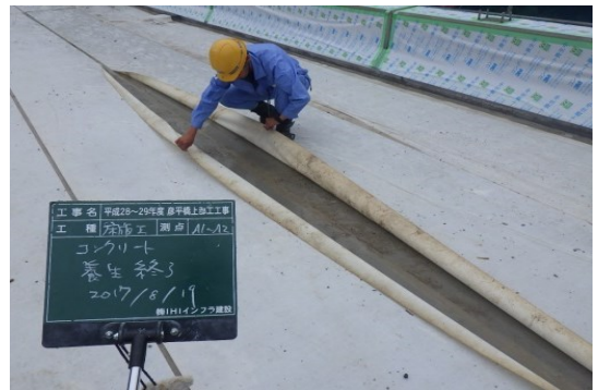
Fig.4.34(e) RC slab was kept wet until 28 days.
