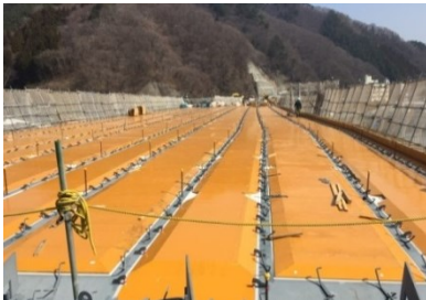
Fig.4.24(d) Permanent and temporary plywood forms for RC slab
