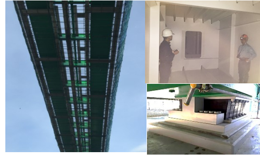
Fig.4.1(b) Continuous box girders and rubber shoe
