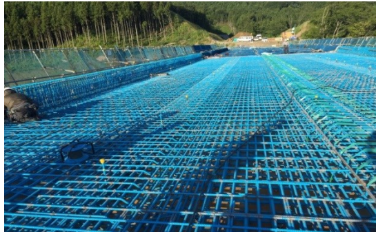
Fig.4.3(a) Epoxy coated reinforcement steel bars
