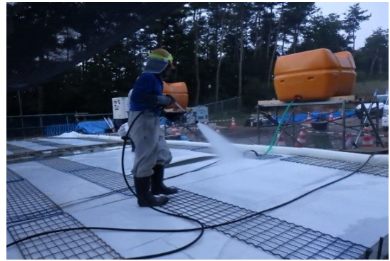
Fig.4.34(c) Spraying water to keep the RC slab wet.
