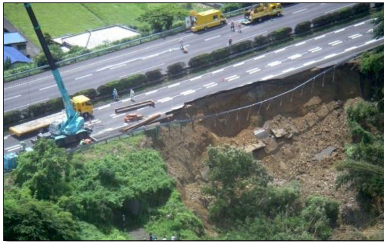
(a) A failure of highway embankment of Tomei expressway in Japan due to Surugawan earthquake
