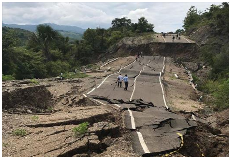
(b). A large settlement of Haliwen-Haekesak road in Indonesia due to landslide after heavy rainfall
