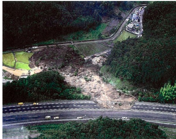
Figure 1.1 Collapse of highway embankment due to heavy rain in Yamaguchi, 2005
