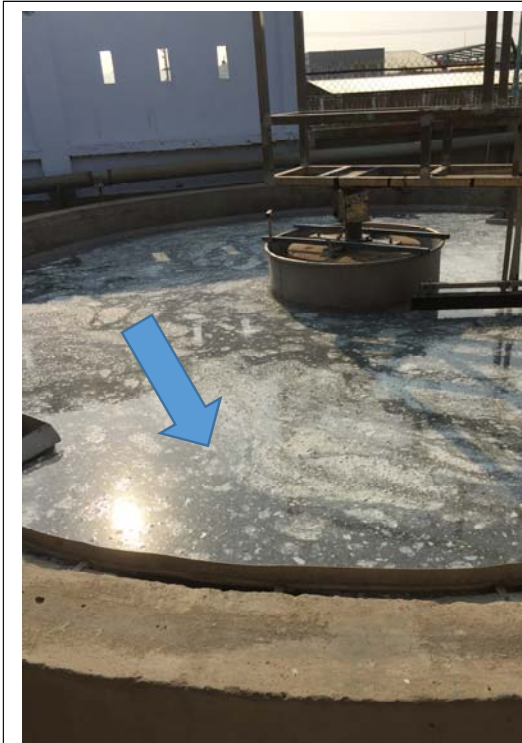
Figure 5.9b. Solid waste drained into wastewater due to refining processing
