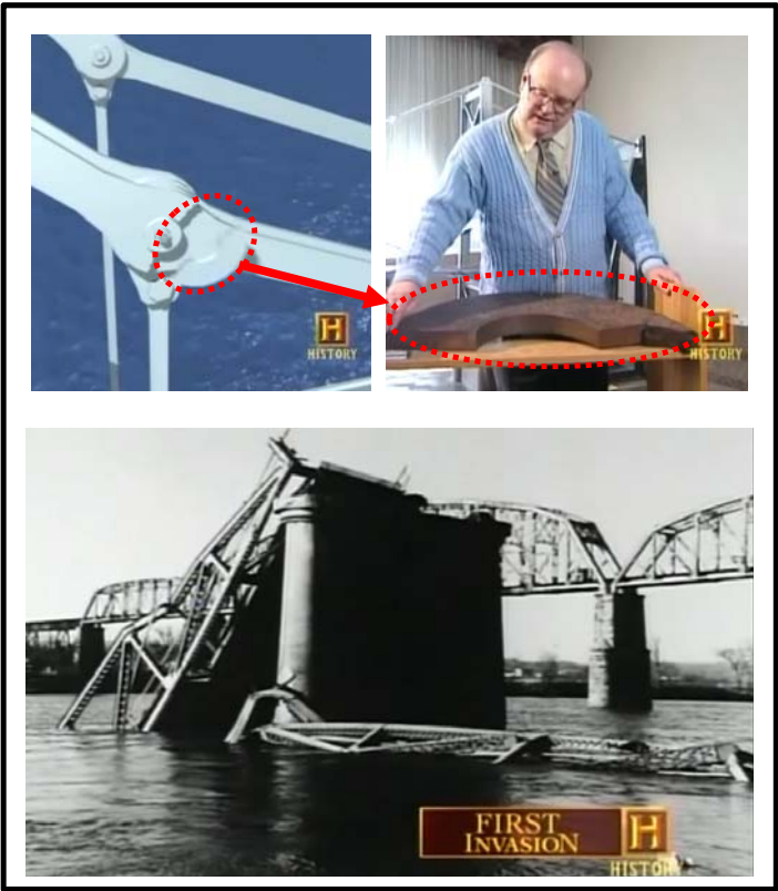
Fig. 1- Collapse of the Silver Bridge caused by of atmospheric corrosion [6].
