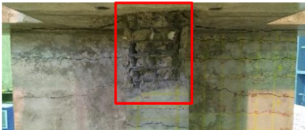
Fig (5.16) Buckling of the longitudinal bars of beam
