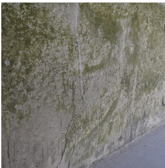
(c) Shimogasawa tunnel
