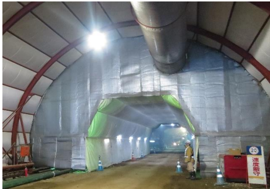
Figure 2.10 Enclosed space used for concreting in some tunnels
