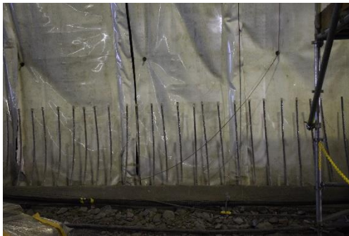
Figure 2.6. Invert close to the tunnel mouth and re-bars
