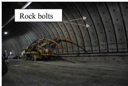
Figure 2.4 steel ring that is installed as a part of first lining
