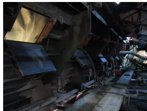
Figure 2.11 Windows provided for concreting at the top part of the formwork
