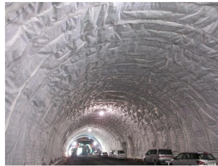
Figure 2.7 tunnel section with laid waterproofing sheet
