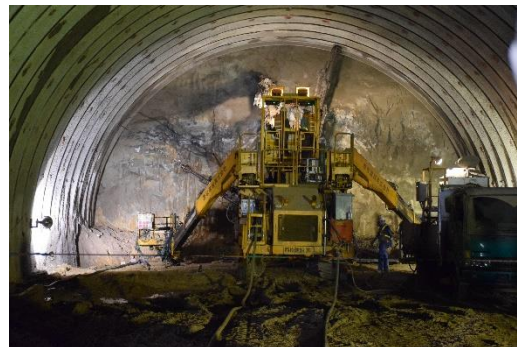
Figure 2.5 Drilling for rock bolts and advancement surface of the tunnel
