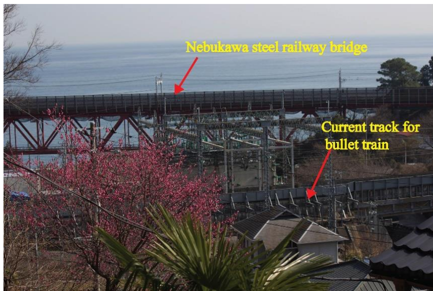
Fig. 5.3 Current track for the high speed train along the Nebukawa region
