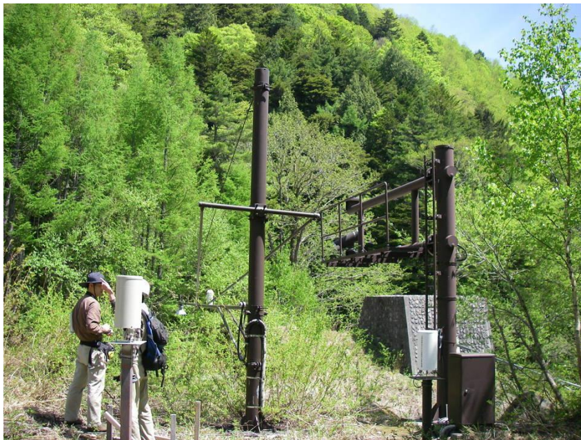
Fig 2.2 Video installation at Kamikami horizawa creek (source: DPRI, Kyoto University, Japan)
