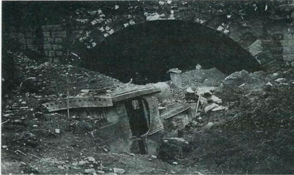
Fig. 5.1 Destruction of Shiraito river debris flow: locomotive of train no. 116 buried near the mouth of Sainome tunnel (JNR 1927)
