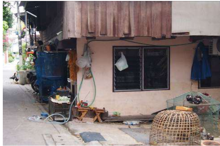
(b) Wood and brick house
