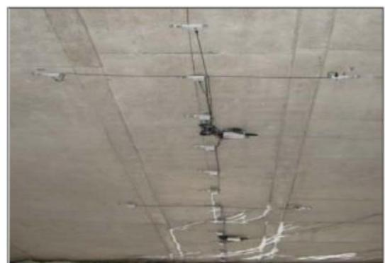
(b) Installed strain sensor
