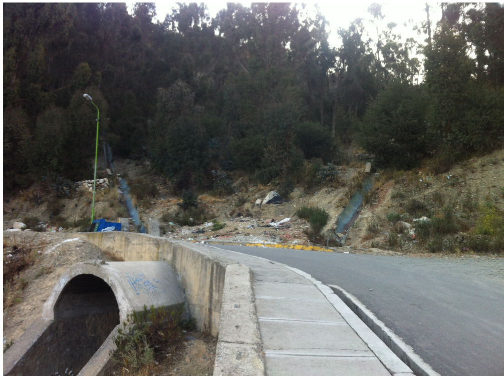
Figure 2-14 River channel crossing a principal avenue of study area
