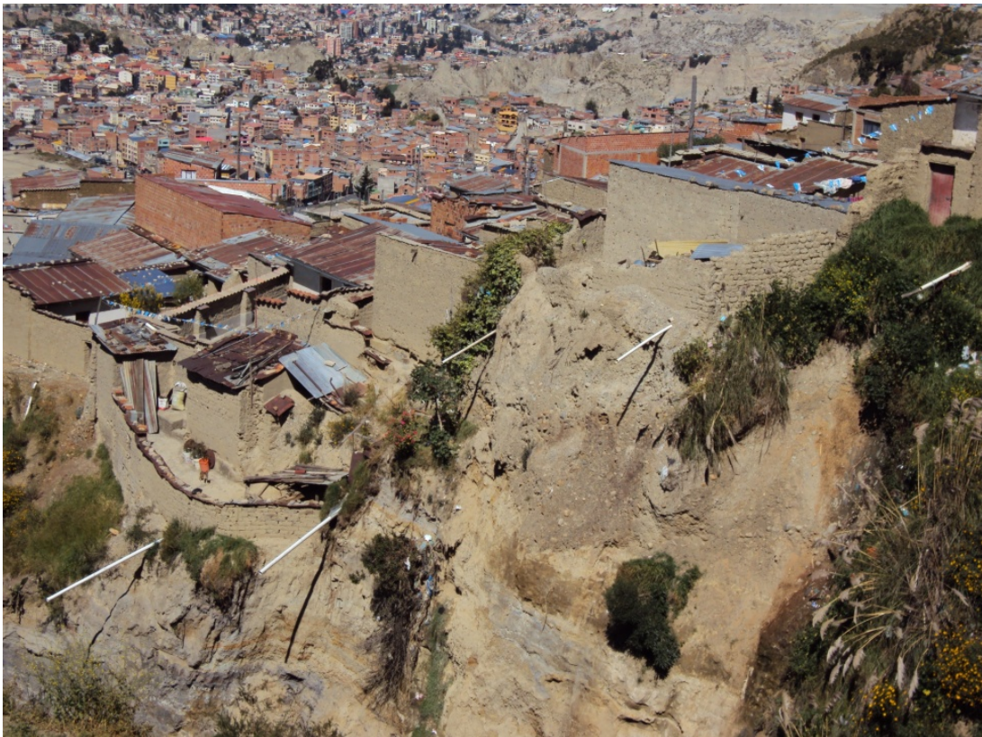
Figure 2-4 Houses located on steep slopes in La Paz
