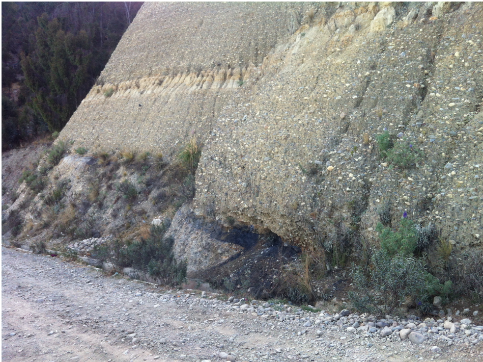
Figure 2-15 Erosion caused by underground river filtrations
