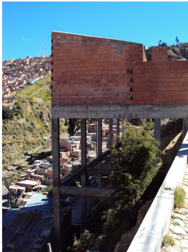
Figure 2-6 Structure of an illegal house in La Paz
