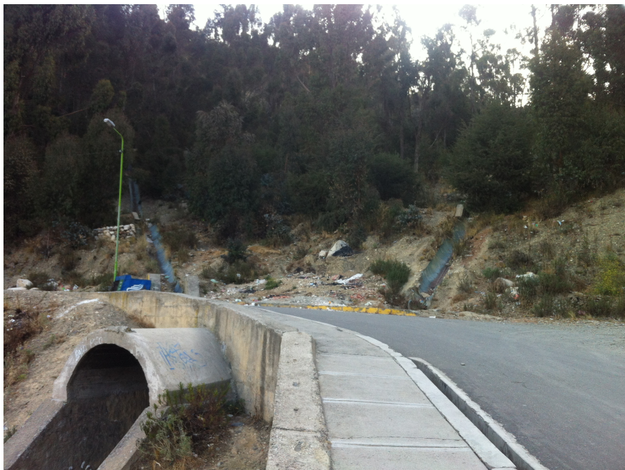
Figure 4-10 Horizontal asphalt street with river channel beneath
