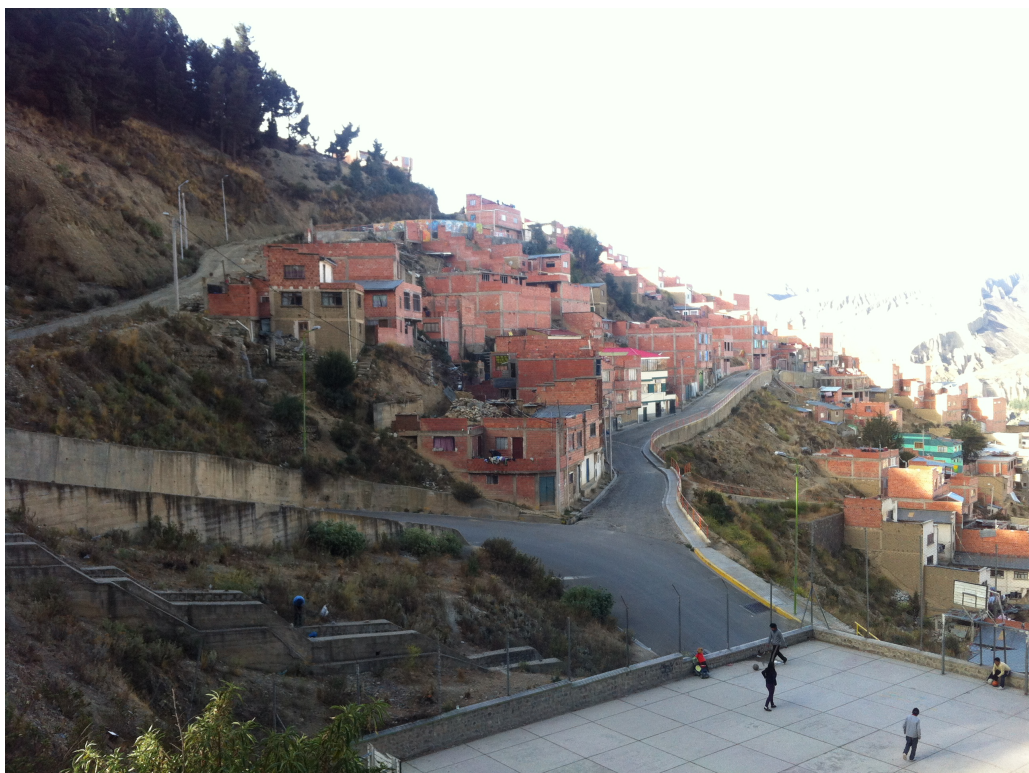
Figure 2-12 General view of Cinco Dedos neighborhood
