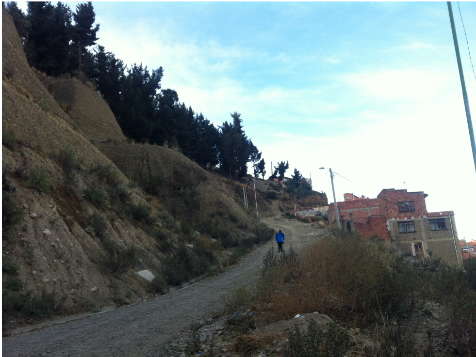
Figure 4-9 Dirt roads on the upper sector of the study area
