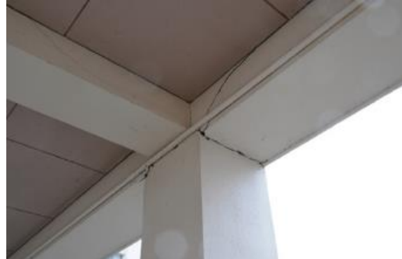
Figure 1-7 Damage in columns [1-9] From left to right: Shear failure and Flexural cracks
