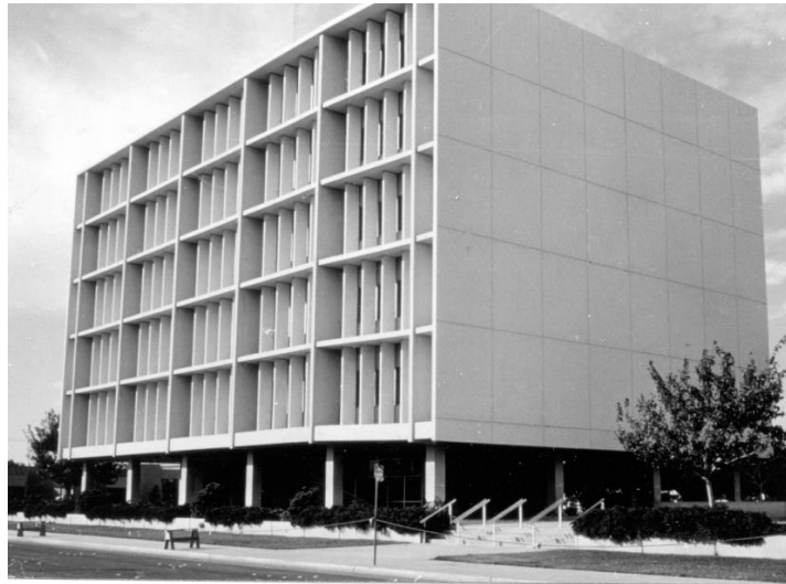
Figure 1-9 Imperial County Service Building Photo by C. Rojahn. Figure 243, U.S. Geological Survey Professional
