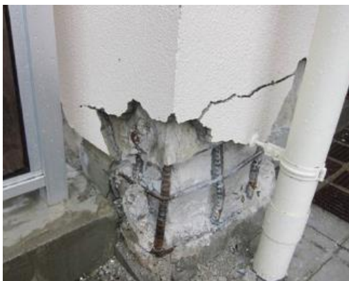
Figure 1-8 Compressive failure From left to right and from up to down: compressive failure in wall [1-10], column designed with the standard low of Japan of 1968, 1974, and 1966 respectively [1-9].
