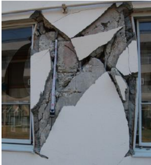
Figure 1-7 Damage in columns [1-9] From left to right: Shear failure and Flexural cracks
