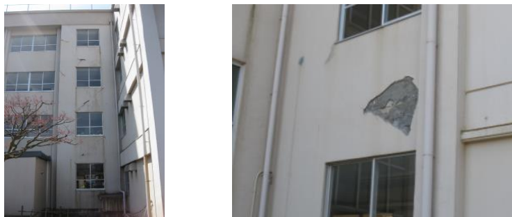
Figure 1-5 Shear cracks in short span beams [1-9]
