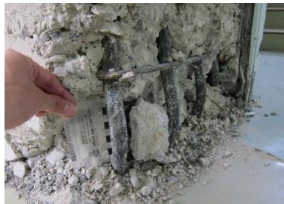
Figure 1-8 Compressive failure From left to right and from up to down: compressive failure in wall [1-10], column designed with the standard low of Japan of 1968, 1974, and 1966 respectively [1-9].
