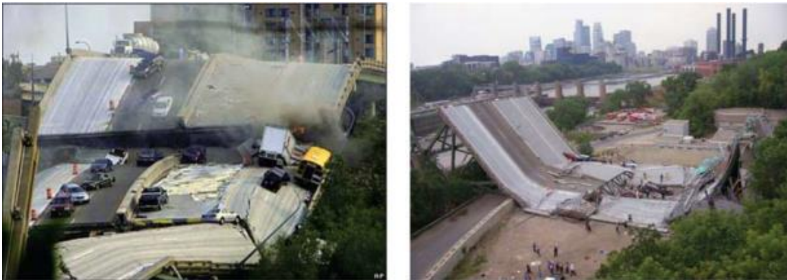
Figure 1.4. The I-35W Bridge collapse [4]
