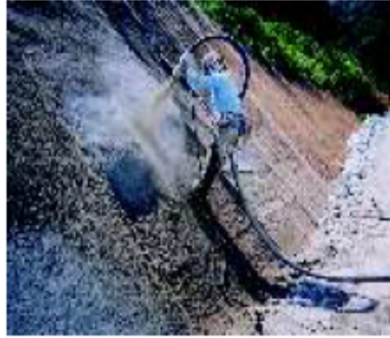
Fig C.7 Application of PVA fiber (Type-A) as shotcreting for slope stabilization 91) .
