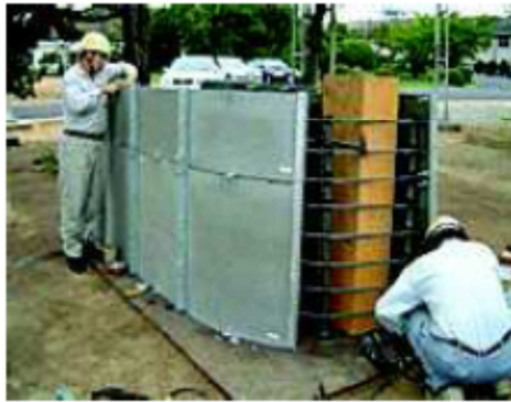
Fig C.5 Application of PVA fiber (Type-A) as permanent framework 91) .
