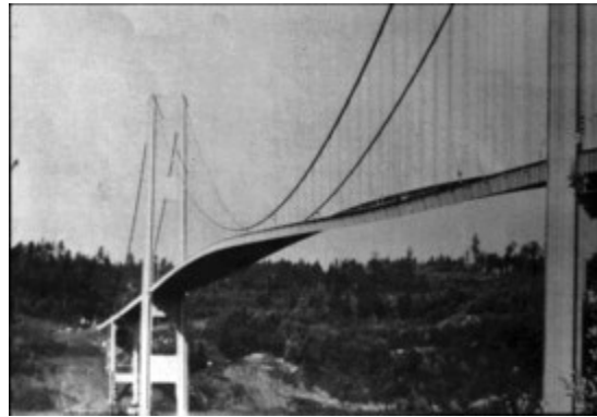
Figure 1.6. The Tacoma Narrows Bridge twisted and vibrated on the day of the collapse [5]
