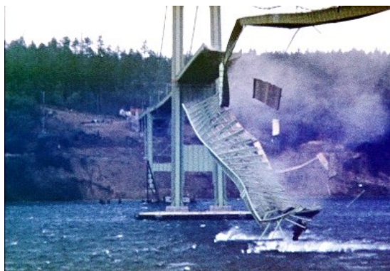
Figure 1.7. The Tacoma Narrows Bridge collapsing [5]
