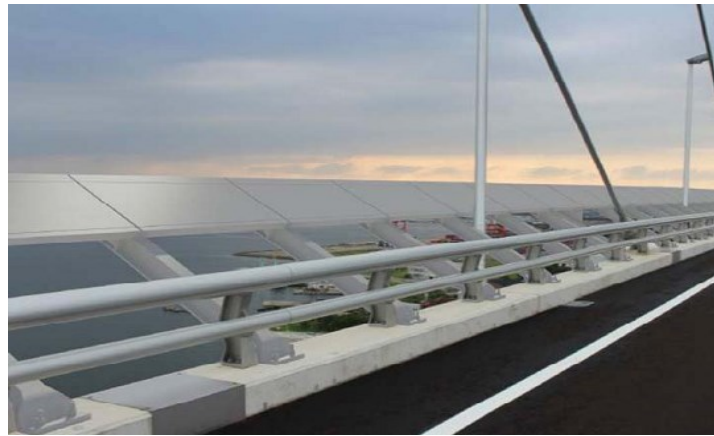
Figure 4.12. Flap (0.22D, 0.29D, 30) installed in the Shin-minato Bridge [7]
