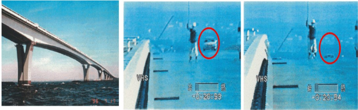
Figure 1.8. Large vortex-induced vibration at the Trans-Tokyo Bay Highway Bridge [6]
