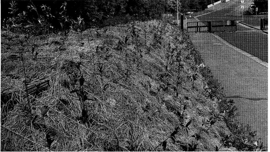
Figure 27. ポット苗植栽後直ちに、地肌が見えない様に、稲藁でマルチングを施す。 Upon planting pot-seedlings, mulching with rice-straws should be made to cover the ground around roots of seedlings.
