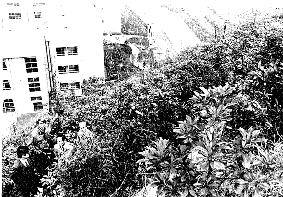
Fig. 12 Successful planting of native trees (EPF) on steep slopes around the Kanagawa Prefectural Kurihama High School, built on re-graded terrain at Yokosuka City.
