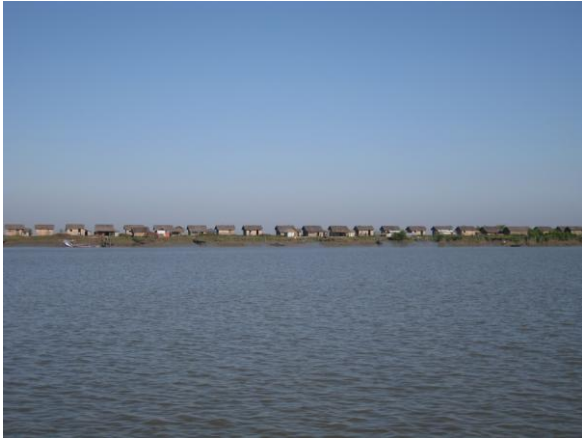
Photo.7.4 Vulnerability of a village along eroded river bank in the Ayeyarwady Mega Delta
