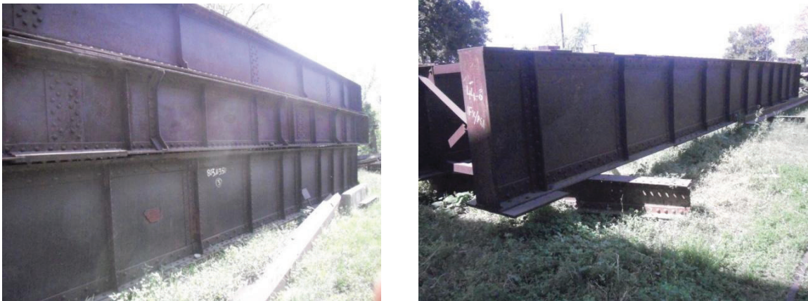
Figure 3.5: The replaced bridged in the yard
