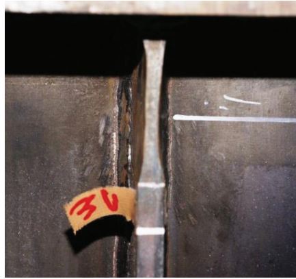
(a) Uniform damage
