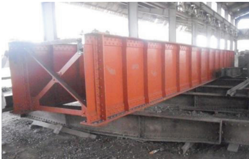
(c) Plate Girder Bridge after retrofitting and repainting
