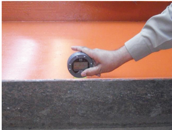
(a) Measurement of paint coating thickness
