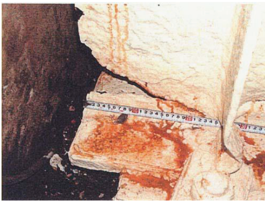
Figure 1.3: Buckling failure of girder due to excessive section lost at bearings
