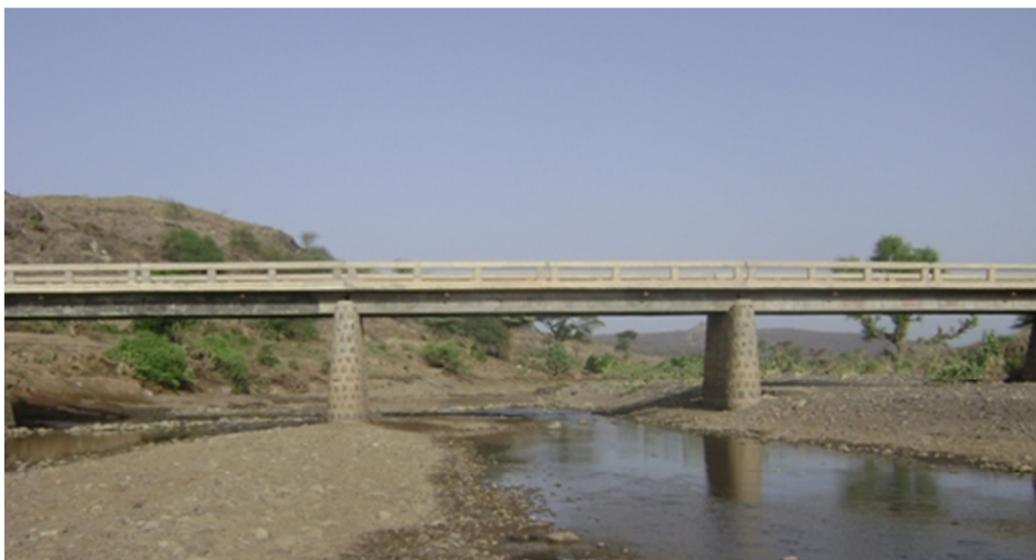
**Fig. 2.6** RC T-girder bridge [2.9]
