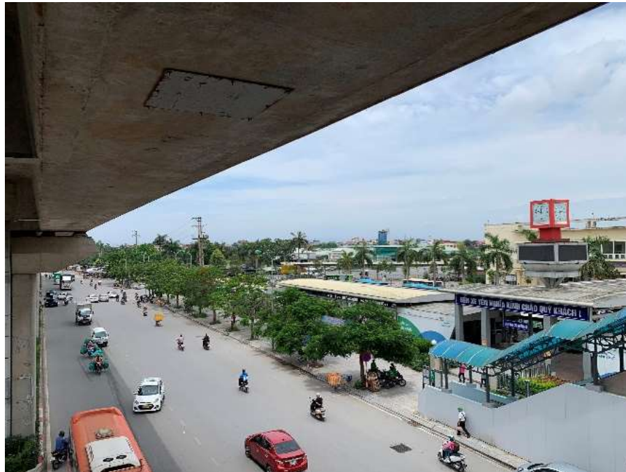
Yen Nghia Station (Station 12) Side exit
