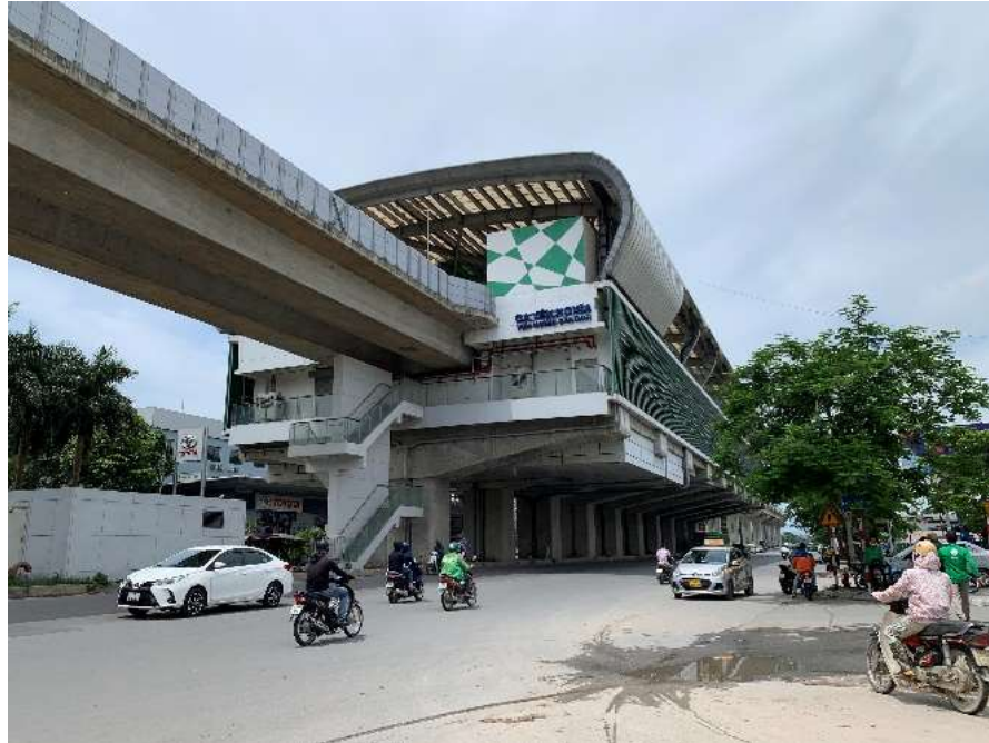
Yen Nghia Station (Station 12) Main exit
