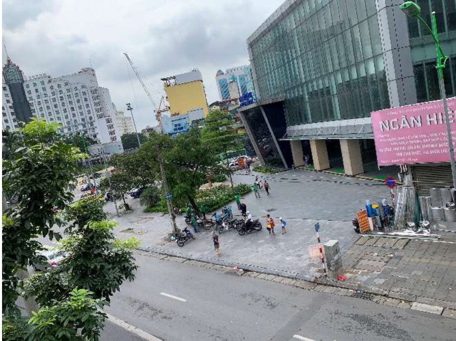
Cat Linh Station (Station 1) Main exit
