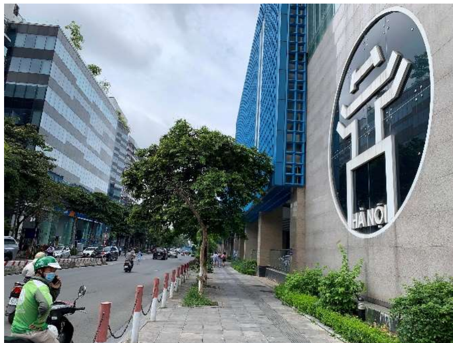
Cat Linh Station (Station 1) Side exit
