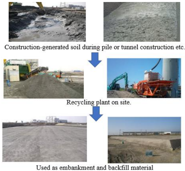
Figure 1.2 Example of recycling construction-generated soil on site
