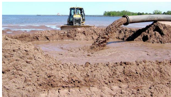
Figure 2.1 Construction-generated soil during pile and tunnel construction
