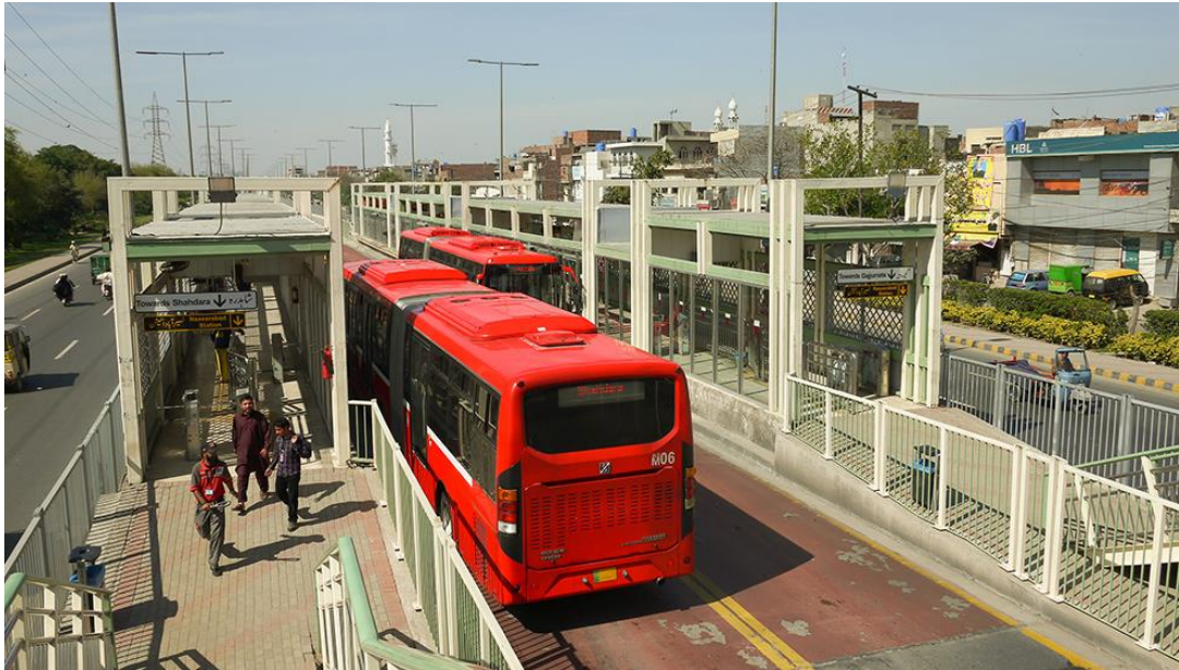
Figure 4.8 BRT station with buses in Lahore
