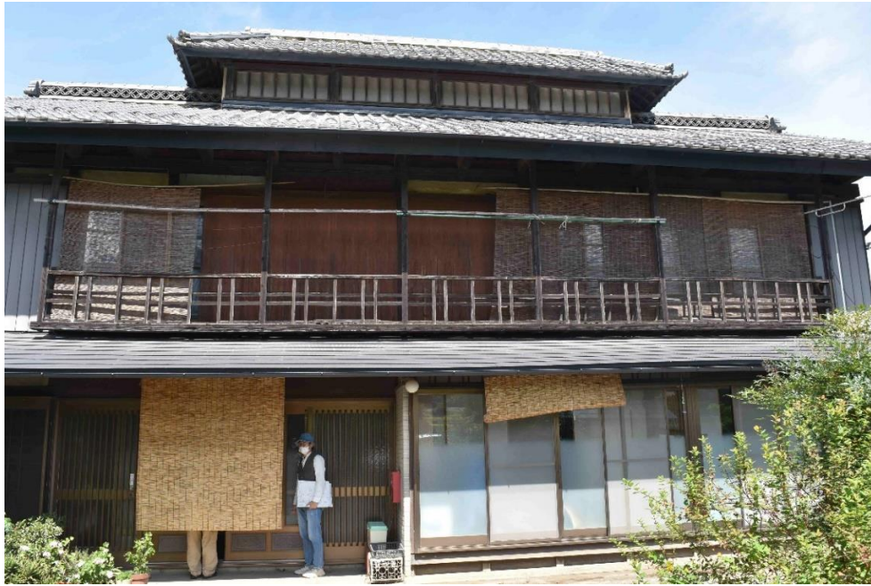
Figure 4-23: Honda Residence omoia with roof ventilation system possessing hipped roof in Ueguri, Agatsuma-gun. (Source: Satoshi Ono. Taken on September 14, 2022.)
