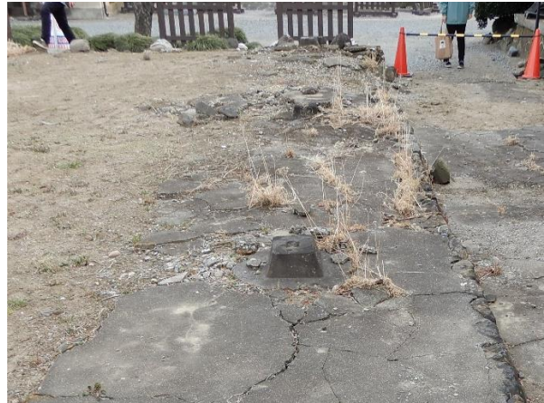
Figure 4-11: Three column stone foundation on the west of remains of shin-sanshitsu . (Taken by Satoshi Ono on January 23, 2022)
