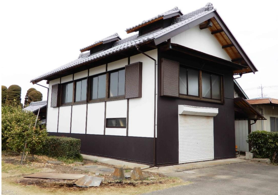
Figure 4-2: Tajima Kameo Residence sanshitsu after repairment.
