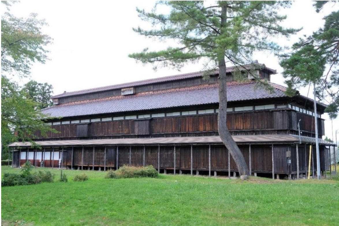
Figure 4-20: No.1 sericulture building in Matsugaoka Reclamation Land.
