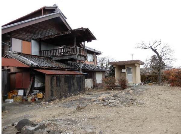
Figure 4-13: Remains of watari-rōka attached to the omoya . (Taken by Satoshi Ono on January 23, 2022)
