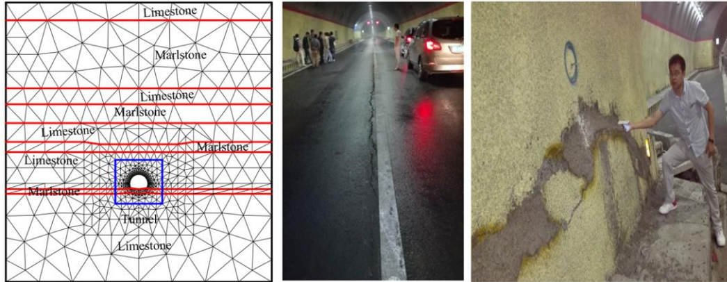
Figure 2-12 Numerical model and lining/pavement cracks in Dugong Ling tunnel due expansive rocks (Liu et al., 2020)
