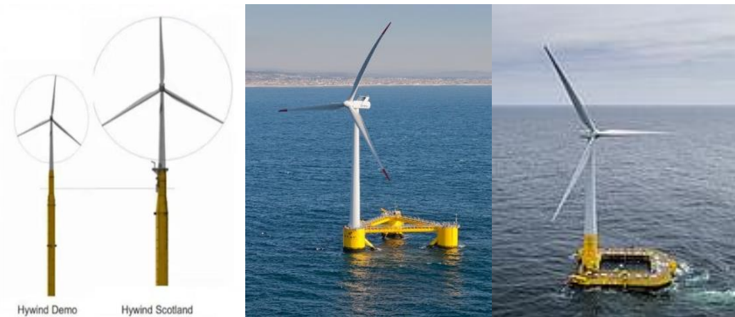
Fig. 1.3 Three types of FOWT (floating offshore wind turbine)
