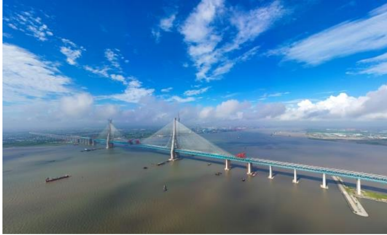
Figure 1.1 An overview of Hutong bridge
