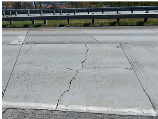
f) Broken concrete slab
