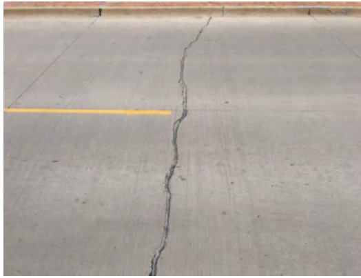
c) Transverse cracking
