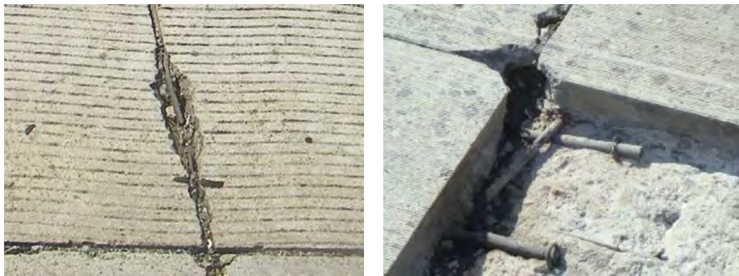
Fig. 1-4 Damage of the sealant and dowel bar of jointed concrete pavements [34].
