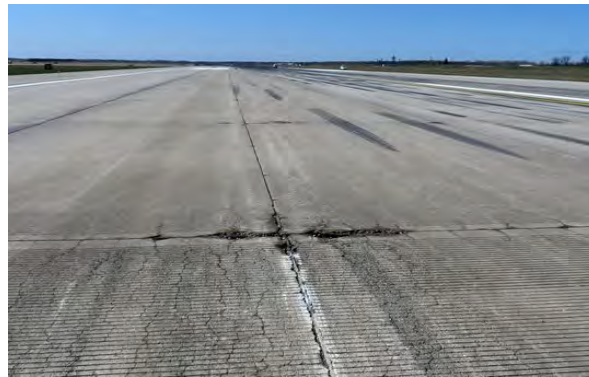
Fig. 1-3 Rainwater in the cracks of the slab [35].
