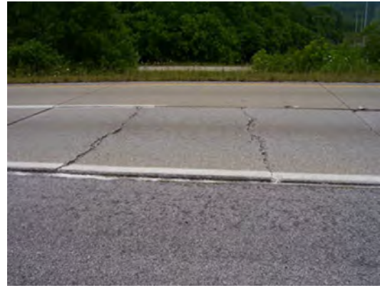
d) Multiple transverse cracking
