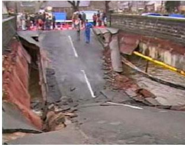
Fig 5.1 Collapse of Ynys-y-Gwas Bridge (From 青木圭一, 2015)
