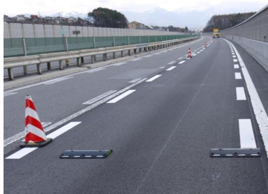
Fig 4.17 Hump Position on the viaduct deck
