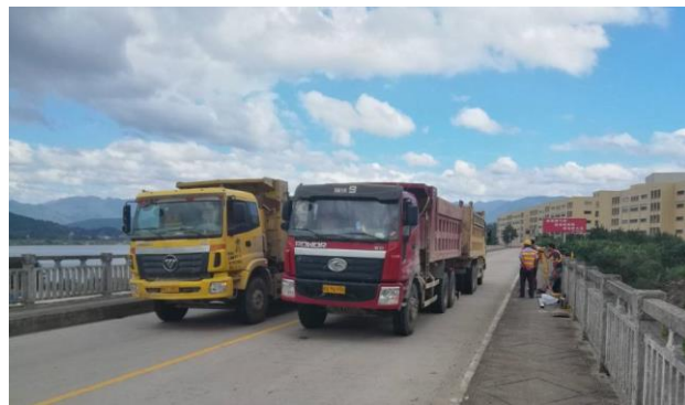
Fig 5.21 Static proof load test
