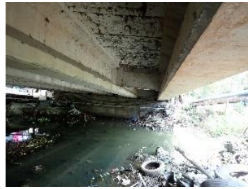
(b) Main girders
