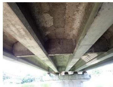
(b) Main girders
