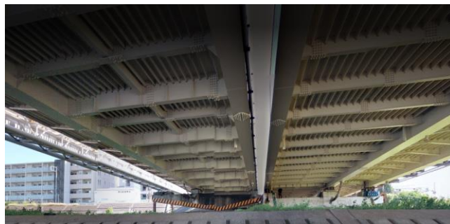
(b) Cross beam and longitudinal rib system
