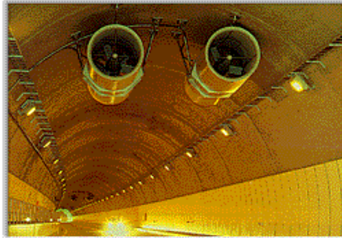
Figure 1.5 Illustration of ventilation system in road tunnel
